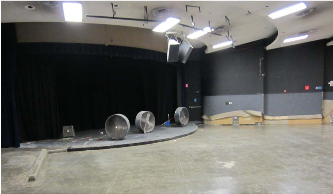
New level concrete floor in old theater
