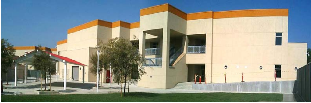
New 2-Story Classroom Building
