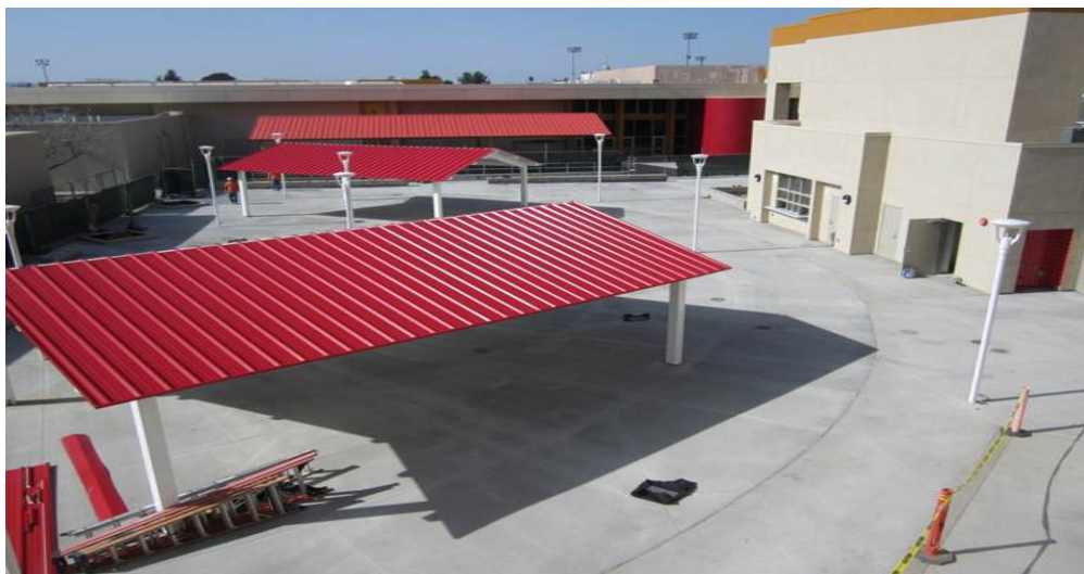
New courtyard with three new shade shelters
