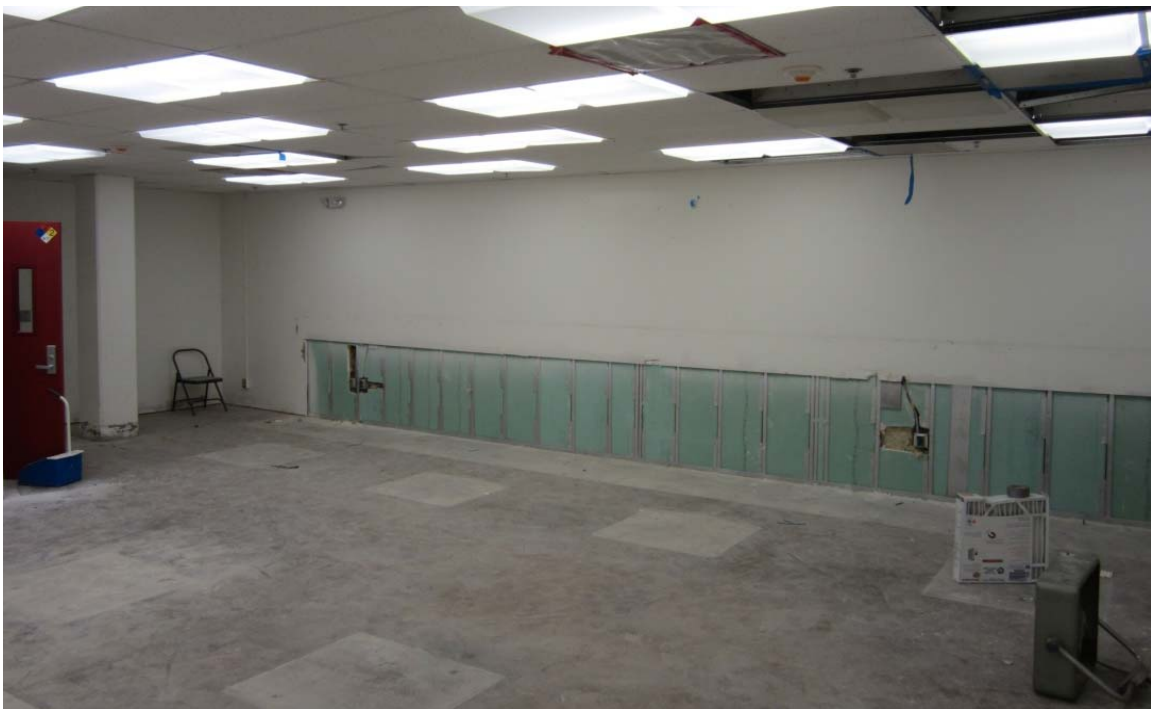
Drywall installed for remodeled classroom
